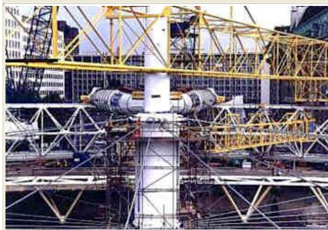
The installation of spoke cables
